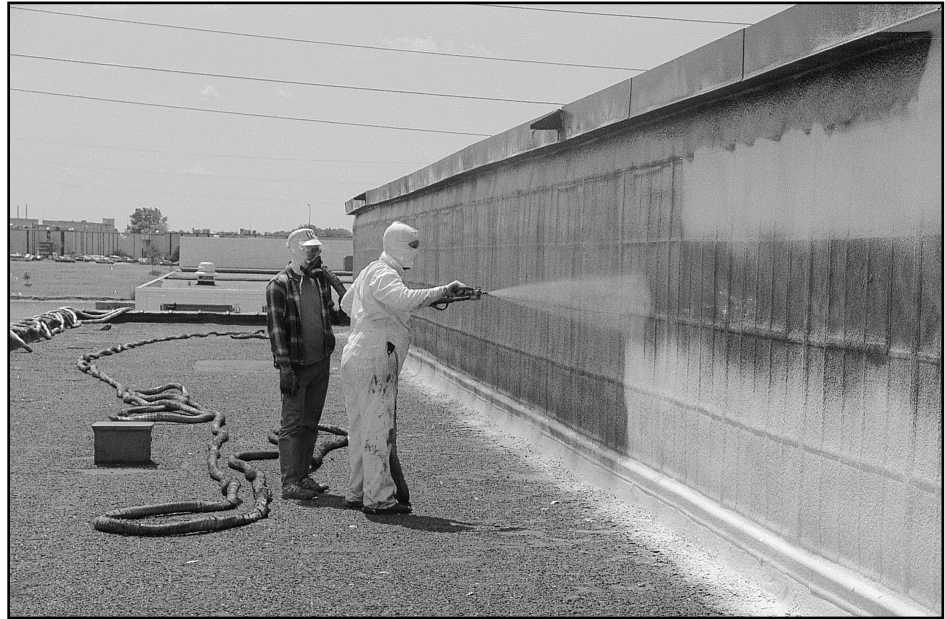
Foam is applied to an exterior wall using Graco Foam-Cat component parts.
